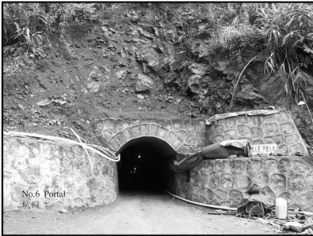
Figure 1 — Highway Mine Portal 6 [4]
